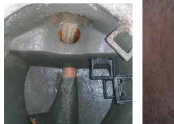
Leak proof and rehabilitated shaft with drop structure
