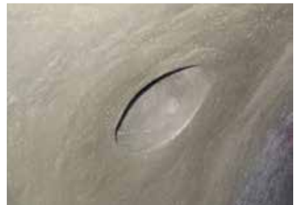
Pipe socket after the rehabilitation
