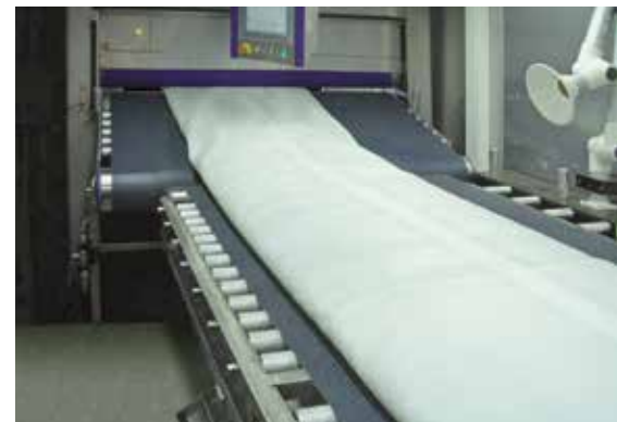
On-site impregnation with the epoxy resin MaxPox®
