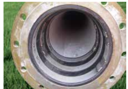
Liner end collar for the connection with the flange mounted before the installation in case of large pipe dimensions
